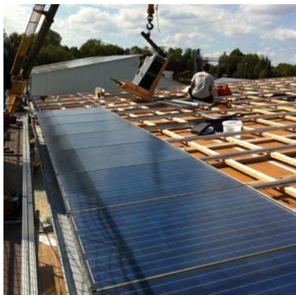
Fastening of modules on the roof battens
