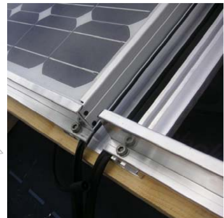
Detail of the fastening system
