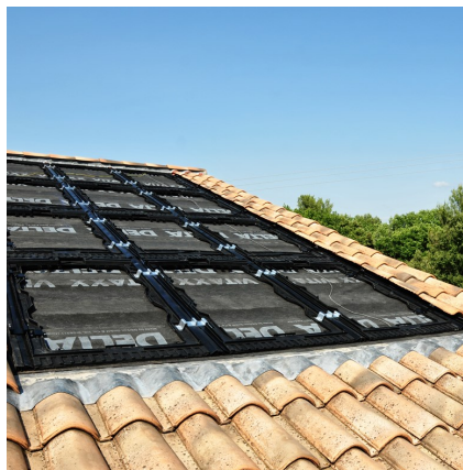
Installation of the mounting system
